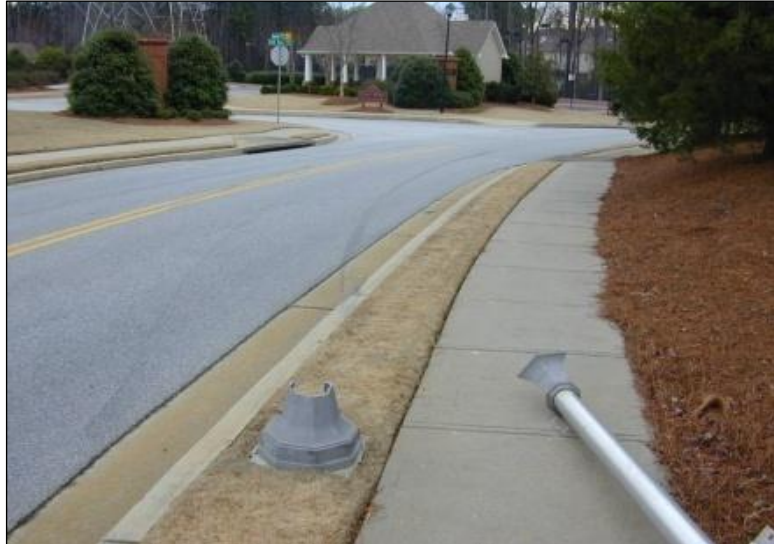
The City of Marietta Police investigated the incident. It was estimated that the vehicle was traveling approximately 40-50MPH in a 25 MPH zone when it crossed lanes and struck the radar sign.
