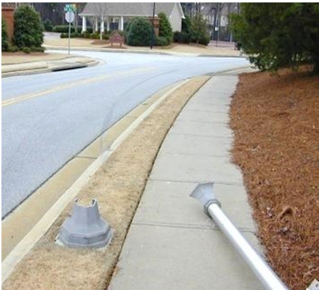
2.) The City of Marietta Police investigated the incident. It was estimated that the vehicle was traveling approximately 40-50MPH in a 25 MPH zone when it crossed lanes and struck the radar speed sign.
