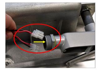
Insert the end of the conduit onto the junction box and tighten the conduit fitting.
